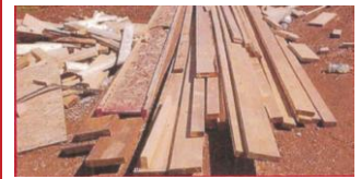
Unsorted pile with cuts & damage – not acceptable
