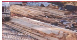
Scattered, mixed with debris – not acceptable
